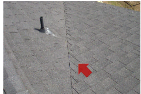
Cut & remove shingles from valleys.
