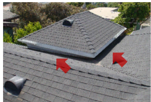
Low slope area has roofing material.
