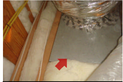
Un-insulated return air filter plenum.
