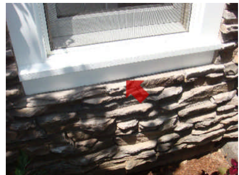
All gaps /voids should be sealed.
