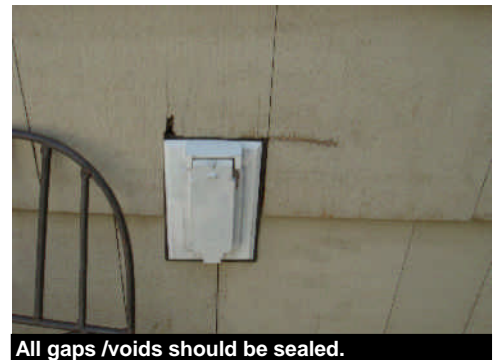
All gaps /voids should be sealed.
